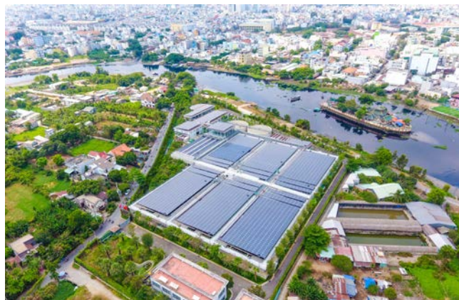
1.4 MW PV Plant Vietnam 🇻🇳
